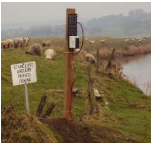
Figure WP4-9: GridStix deployment at Cow Bridge
